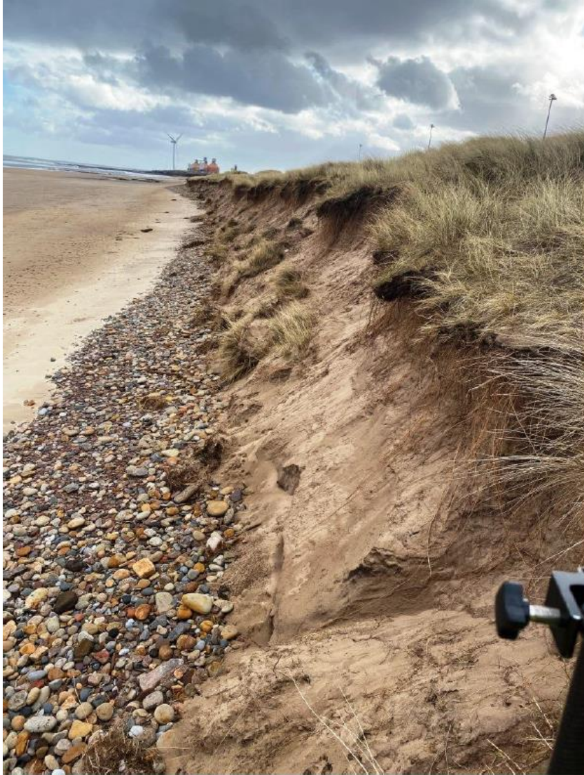
Plate 1 Section of erosion along Cambois bay
